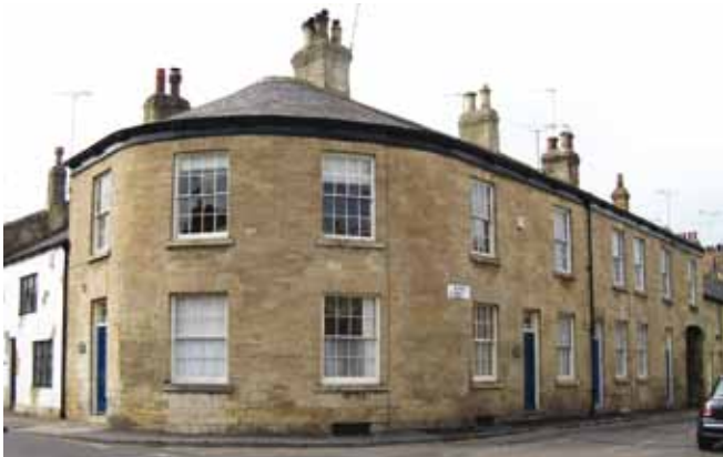
The curved frontage of these buildings is a unique feature and creates an interesting streetscape. Other details such as the window forms, doors and chimneys contribute to the character of the properties and all such details are important.
