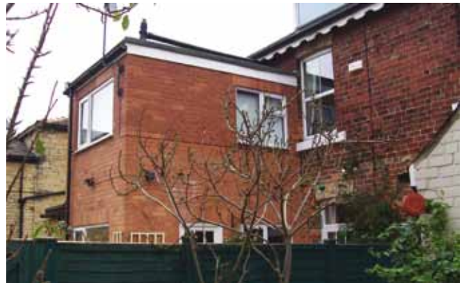
Care should be taken to ensure that windows are positioned to avoid overlooking neighbouring gardens.
