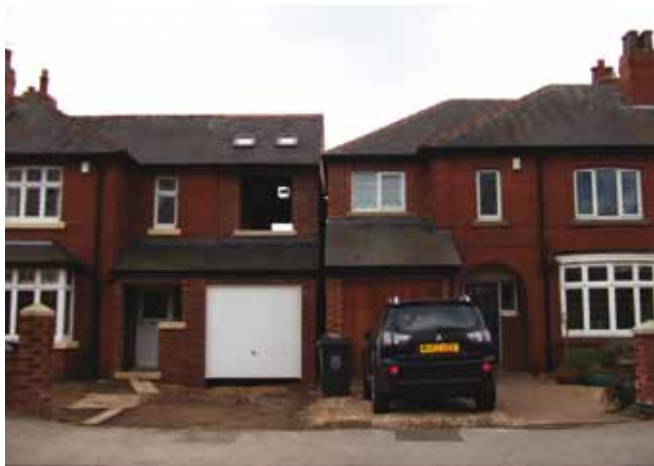
These two side extensions are built over the driveways of the houses and have wholly closed the gap between the two buildings.
