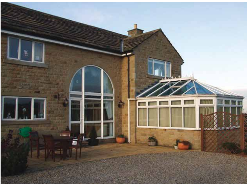
The use of obscure glazed or solid side panels prevents the neighbouring garden being directly overlooked.
